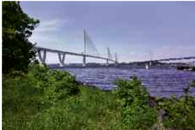
Forth Replacement Crossing bei Edinburgh © Transport Scotland
