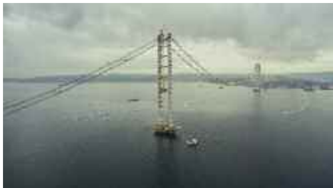
Montage der Izmit Bay Crossing Bridge © Maurer AG
